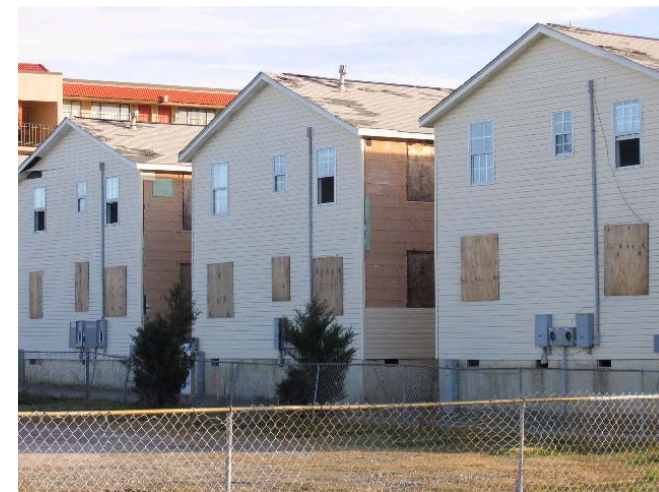
Buildings boarded up in the CBD
